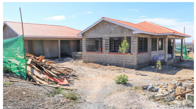
Rumuruti seed production center under construction
